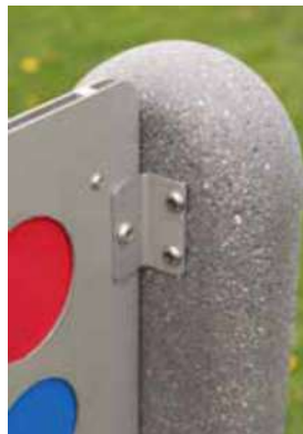
Stainless steel tamper resistant screws used to secure the game to the concrete supports.
